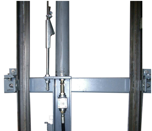
Image 19. Strut fixing.
